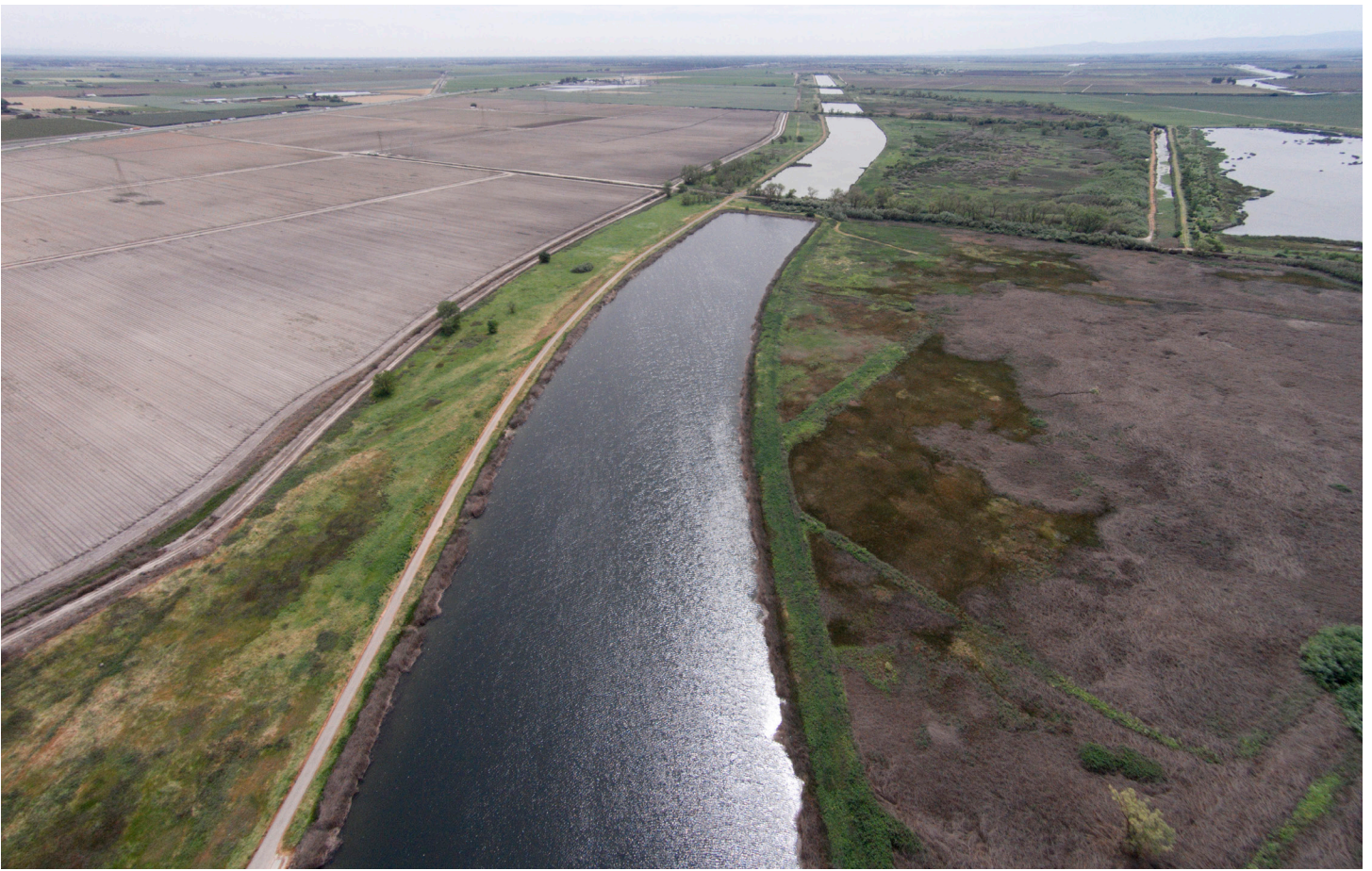
Figure 4 Water infrastructure that was never realized: Ponds #9–13 of the White Slough Wildlife Area. These ponds are the borrow pits from the building of the nearby I-5 embankment. The ponds were dug in this linear fashion to strategically begin excavation of the proposed Delta peripheral canal. When the peripheral canal was voted down in 1982, these lands were retained by the state of California and turned over to the California Department of Fish and Wildlife for management under “interim” status. Today, as part of the White Slough Wildlife Area, they still retain this interim status. Fishing, hunting, wildlife viewing, and a variety of other recreational activities occur within the area. Photo: Brett Milligan.
