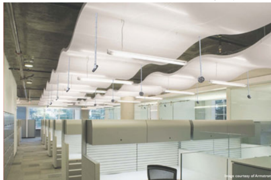
(c) Concept integrating small fans with the ceiling to offer point-source air movement throughout a re-configureable, open-plan workspace.
