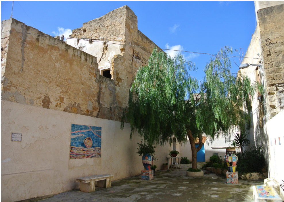
Figure 6. Renovated courtyard with whitewashed walls and ceramic tiles.
