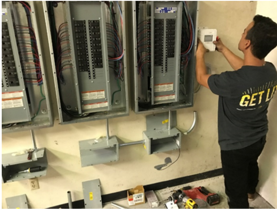
Figure 65: Franco Center Monitoring Equipment Installation
