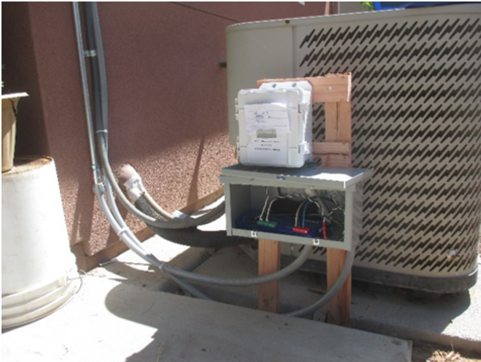
Figure 68: Parksdale 2 Typical Dwelling Unit Monitoring Equipment Installation
