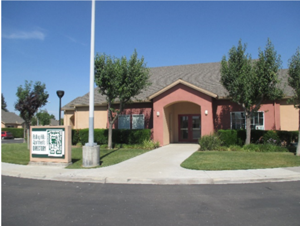
Exterior view of Rolling Hills Community Center building.
