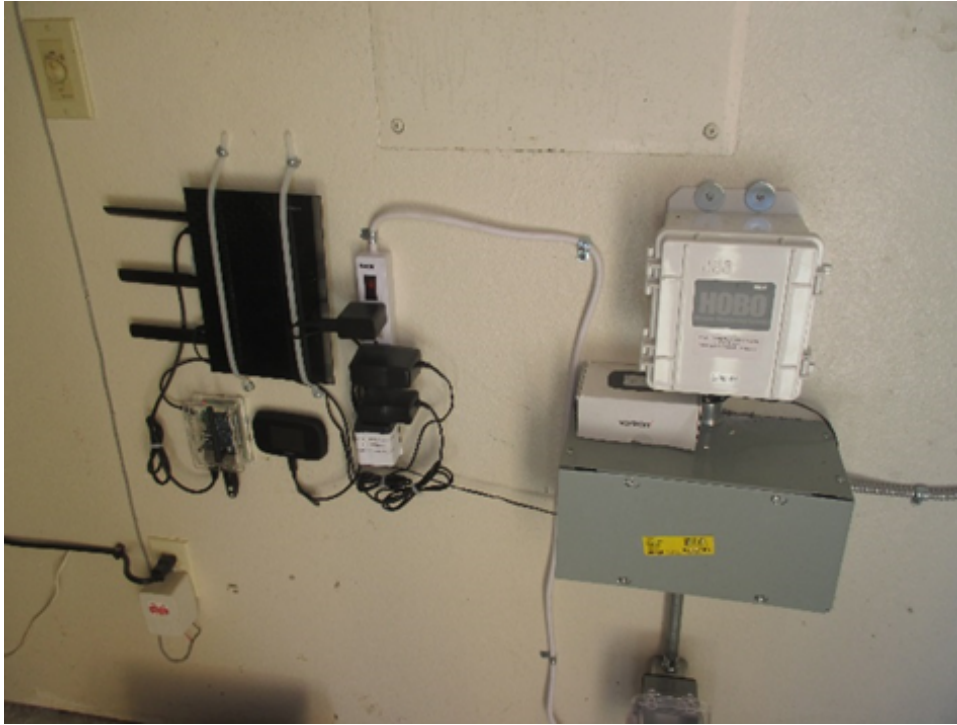
Figure 66: Rolling Hills Monitoring Equipment Installation
