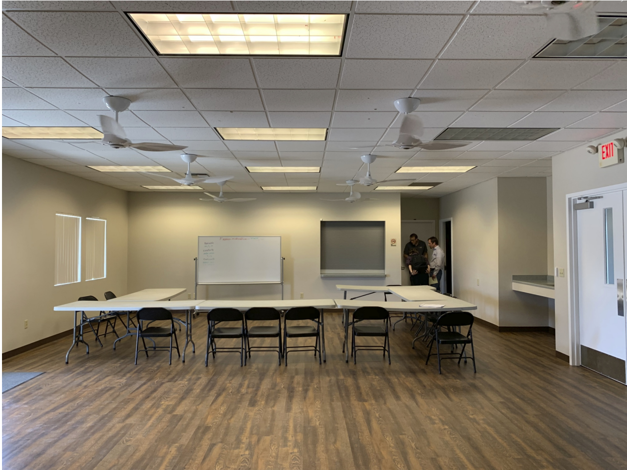
Figure 79: Rolling Hills community room with ceiling fans installed
