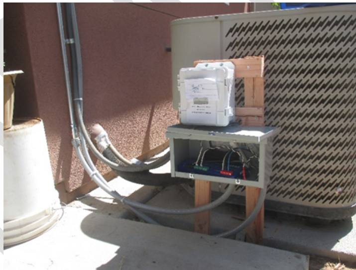
Figure 6: Parksdale 2 Typical Dwelling Unit Monitoring Equipment Installation
