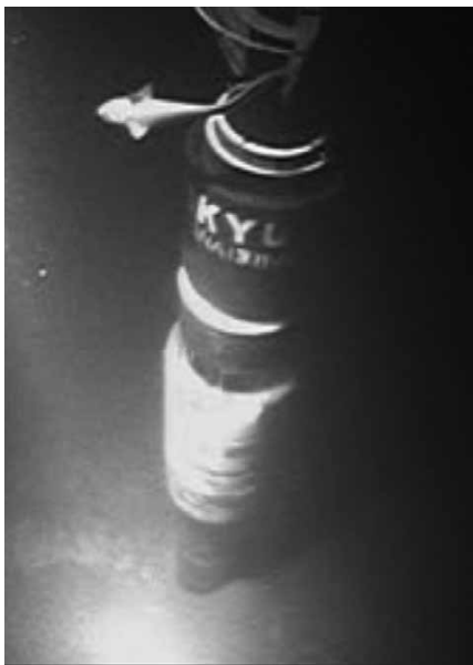
Figure 3. Wellhead for the temperature observatory installed in a borehole on July 7, 2012, in the area above the slip region of the 2011 Tōhoku-Oki earthquake. The seafloor is at a depth of about 6,900 m. Photo courtesy of JAMSTEC
