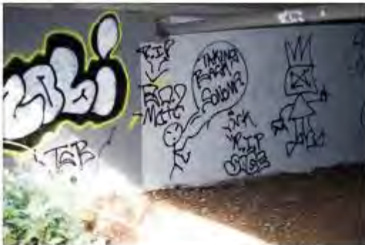
Graffiti under bridge
