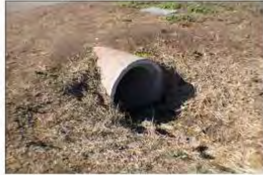
transect 4 set point back shot culvert drain location
