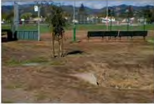
transect 4 set point back shot culvert drain location II
