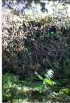
transect 3 bank erosion and overgrown veg
