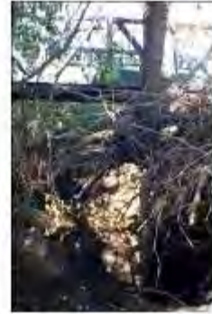
transect 4 left bank bottom root erosion tree hanging on edge of bank
