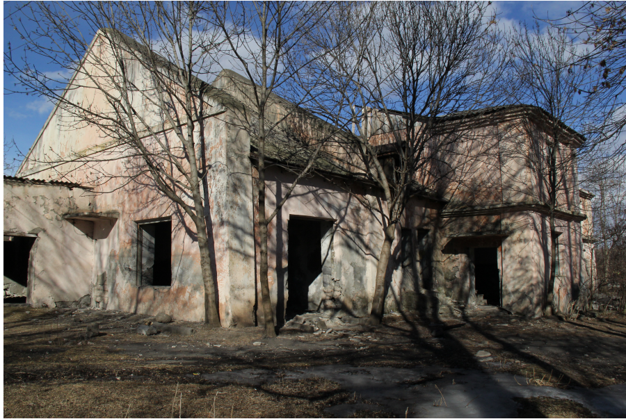
Photograph 4: The abandoned dairy school in Karabulakh village (2014).
