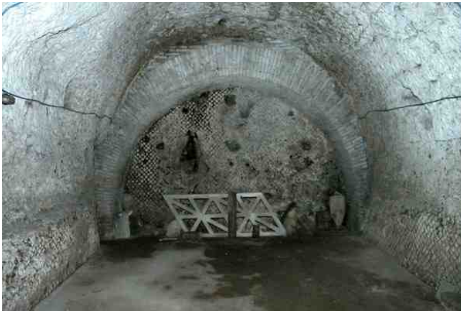
Figure 5.3. Surviving substructures of the cavea: digital composite The Pompey Project ( http://www.pompey.cch.kcl.ac.uk/Site_Documentation.htm , last accessed 1 May 2011)
