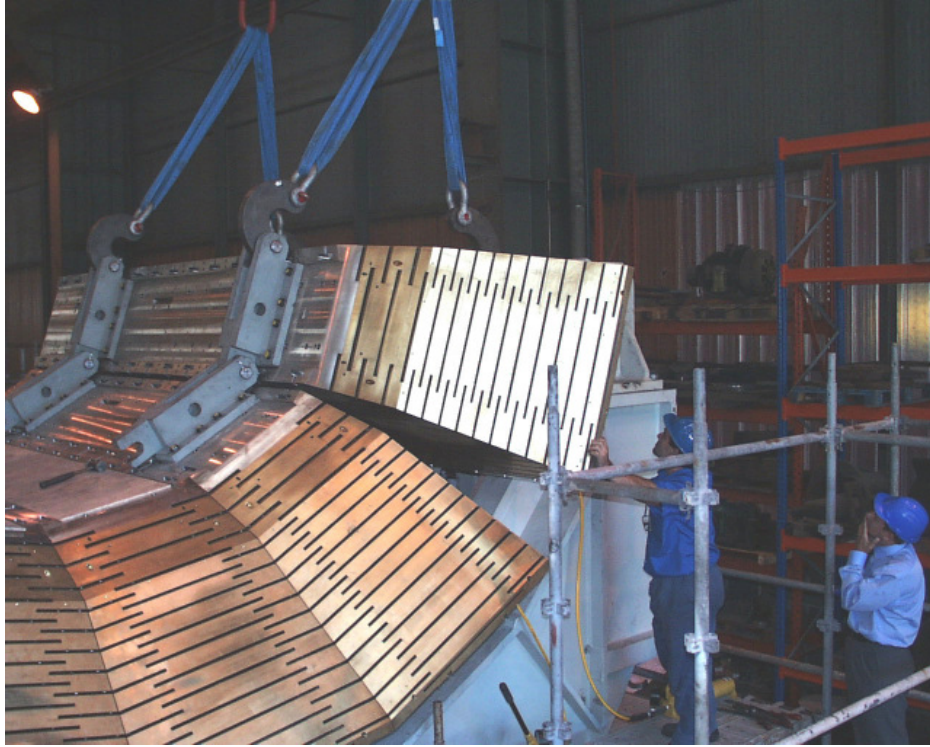
Figure 28: Assembly of the 7th wedge of the HCAL during a hot day of August in 2000. Courtesy of L. Veillet.
