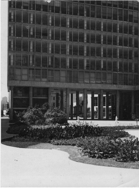
Fig. 10. Ministry of Education and Health, south facade, Rio de Janeiro, ca. 1945. Photograph by Marcel Gautherot. Courtesy of Arquivo do IPHAN, Rio de Janeiro.
