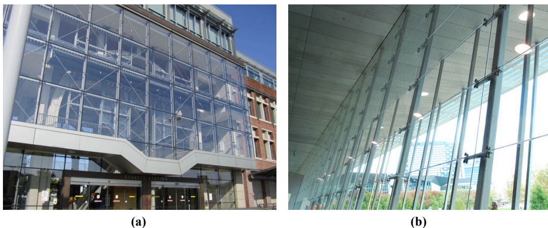
Figure 1.2. Examples of spider glazing: (a) Everett Station (CC image courtesy of SounderBruce on Flickr), and at Melbourne Exhibition Center Station (CC image courtesy of Ding YangYang on WikiCommons)
