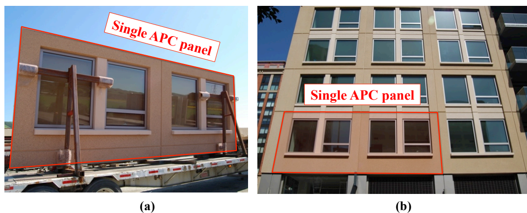
Figure 1.3. Example of APC panels (a) during transportation and (b) installed on a building (Images courtesy of Mark Hildebrand)
