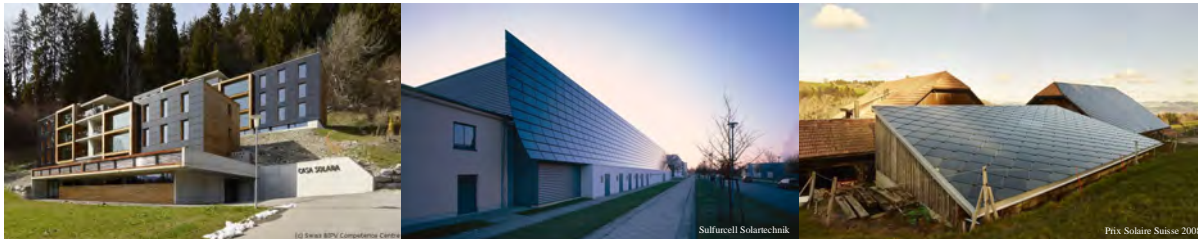
Figure 5.2: Rooftop and BIPV system for a variety of building types [63].
