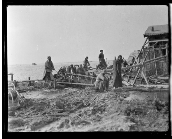
Figure 3. Flooded area being pumped by hand, Tianjin, 1918.
