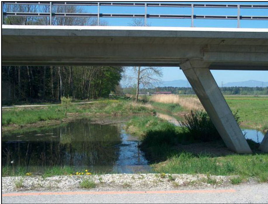
Figure 5. The T10 between Morat and Neuchâtel cuts through important wildlife corridors. Appropriate mitigation measures such as this bridge replacing a culvert were taken. Photo courtesy of Marguerite Trocmé.
