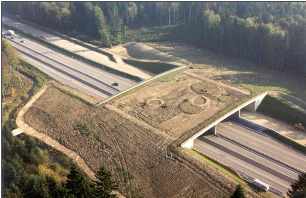
Figure 4. Neu-Ischalg in Canton Bern. The 50-m-wide overpass spans both the existing highway and a new high-speed train line. Photo courtesy of Tiefbauamt canton Bern.
