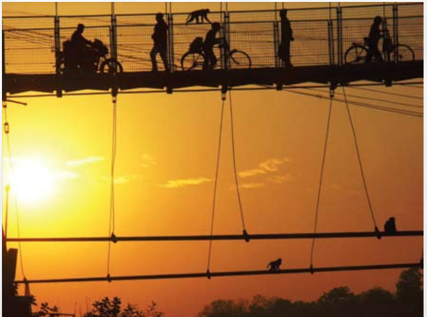
Pedestrian Bridge , photograph, Parker Duncan, MPH, Class of 2008
