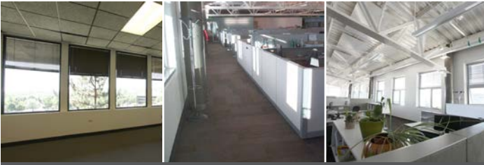
Figure 5-3. NREL's daylighting solution and result of occupant engagement process Left: NREL's previous solution: manual blinds and lights on Middle: NREL's RSF solution: no blinds on the lower glass but some hours of direct sun Right: Occupant engagement process result: glare screens used only where and when needed
