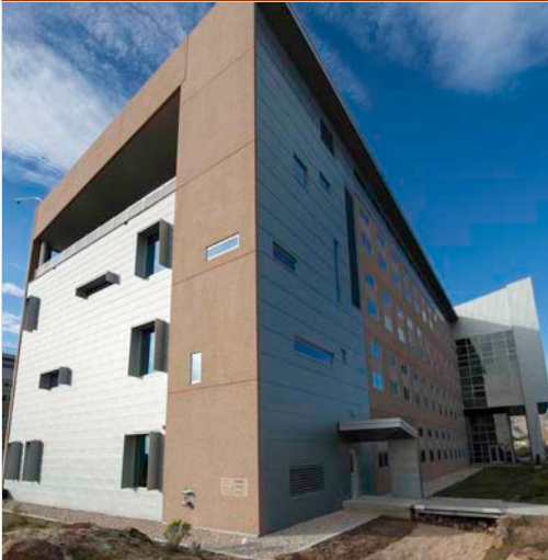
Photo by Dennis Schroeder, NREL 23186
