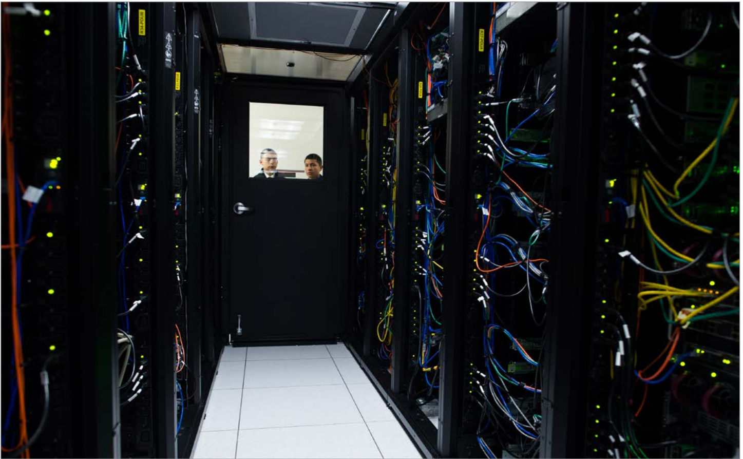
Figure 4-3. Tidying cable can improve airflow problems
