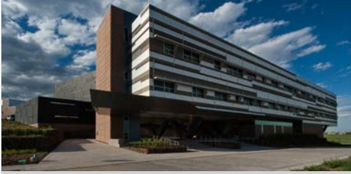
Photo by Dennis Schroeder, NREL 25933
