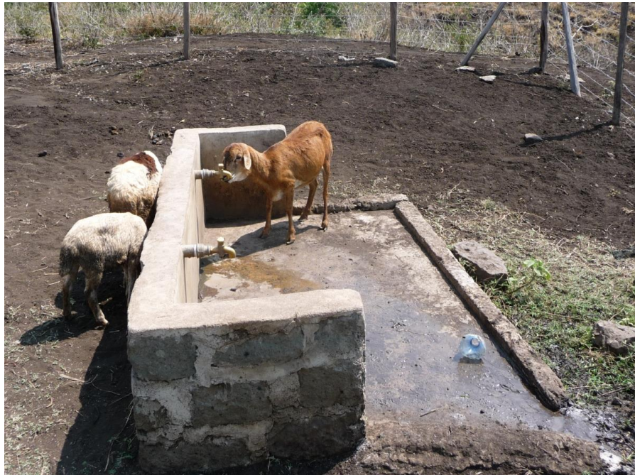
Figure 2. One of the engineering systems in Namerokamano being re-contaminated by a goat and a plastic-bottle funnel stored on the ground.
