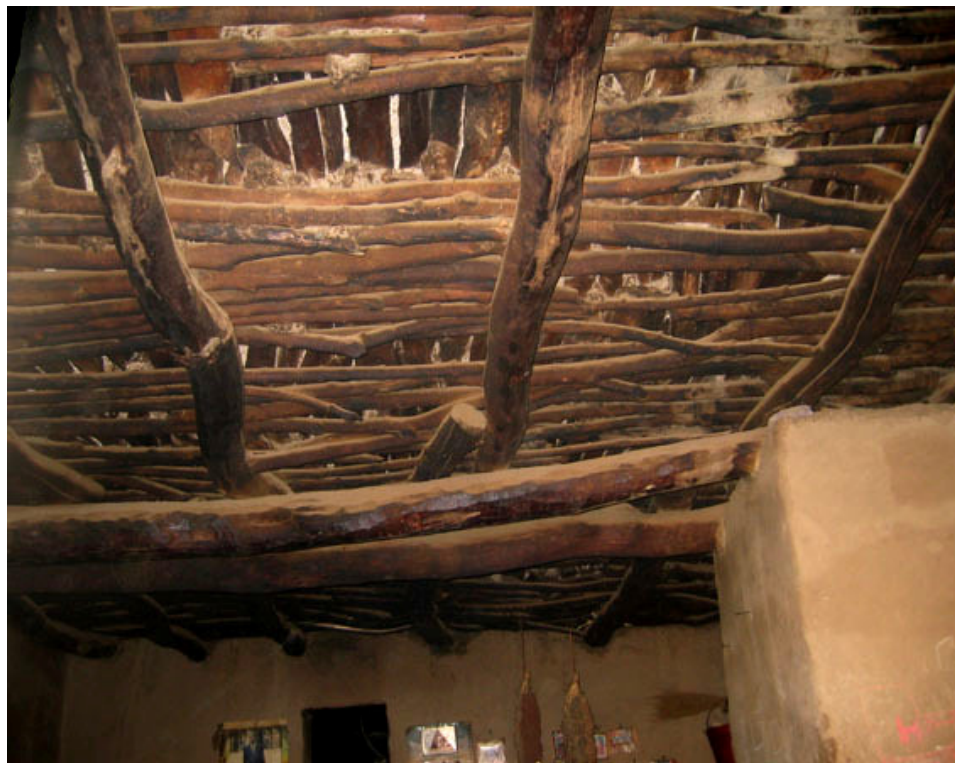
Figure 5.1. A traditional wood-beamed roof from a house in the Sahel, a transition zone along the southern edge of the Sahara desert in Africa. 1 The construction technique here is very similar to that of houses in the ancient Near East, including during the Iron II period. Note the load-bearing wall on the right, which shortens the required length of the main girders running left-right in the photo.
