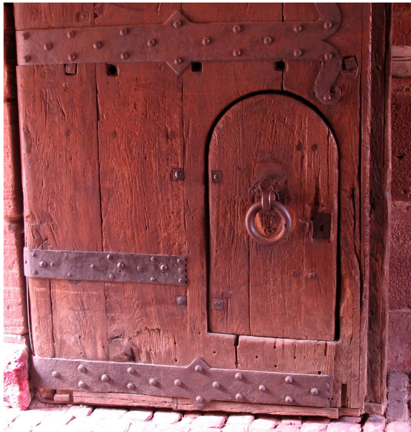
Figure 4.5. A small wicket door built into a gate leaf (here, in a medieval castle) for pedestrian traffic. Heidelberg Castle, Germany. 1
