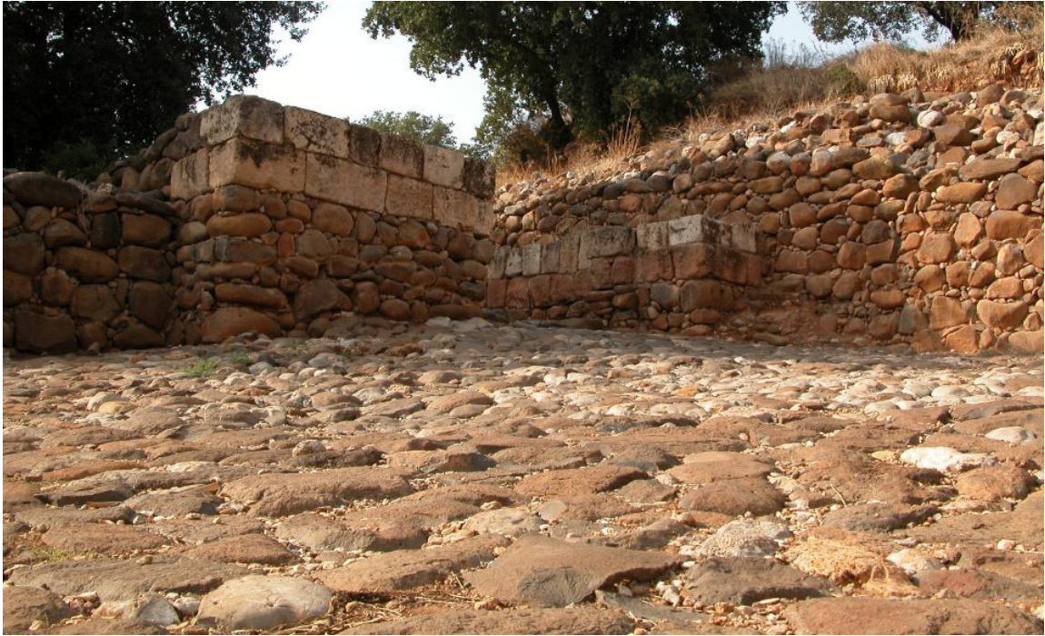
Figure 6.1. The cobblestone-paved outer plaza at Tel Dan’s Iron Age gate, leading to the outer (simple) gate. 1
