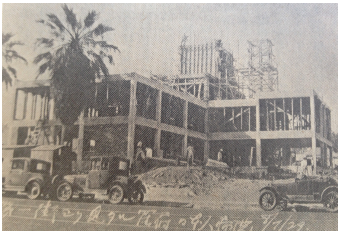
Image 2.4 Construction the new Japanese Hospital 105
