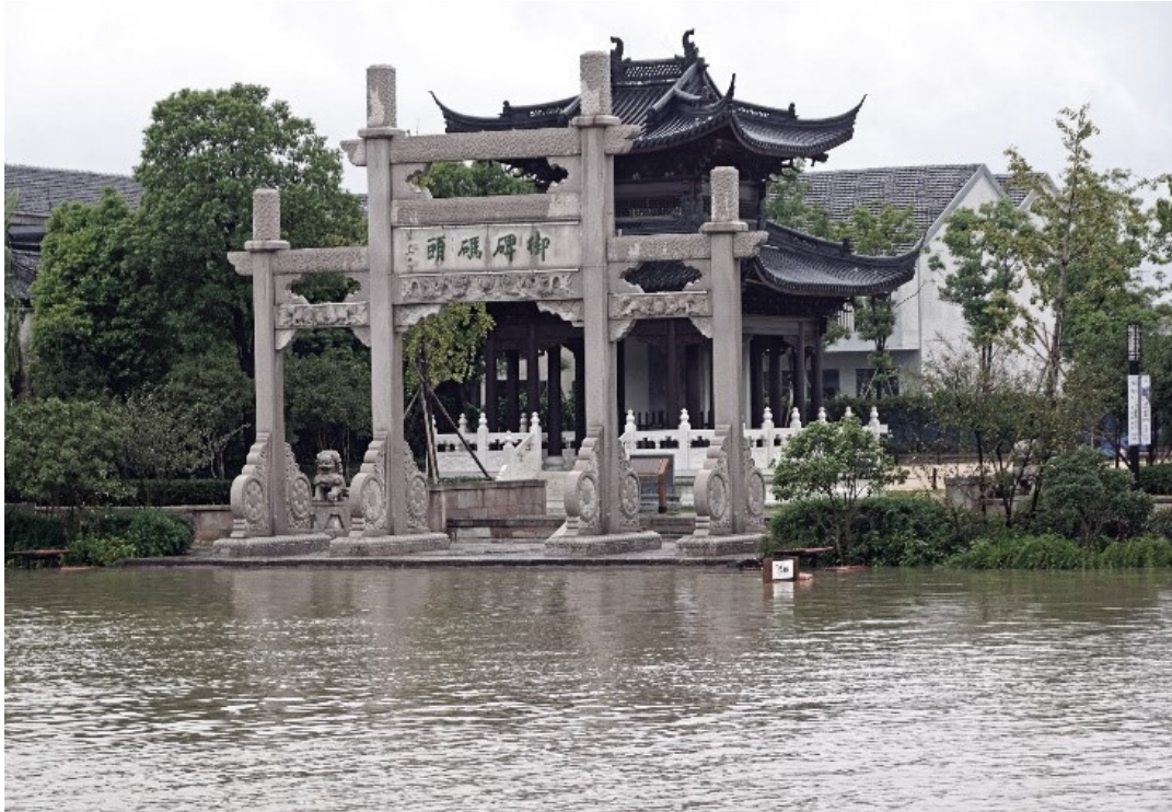
Fig 30 – Yong Village 01, flooding day, provided by the City of Hangzhou, 2022
