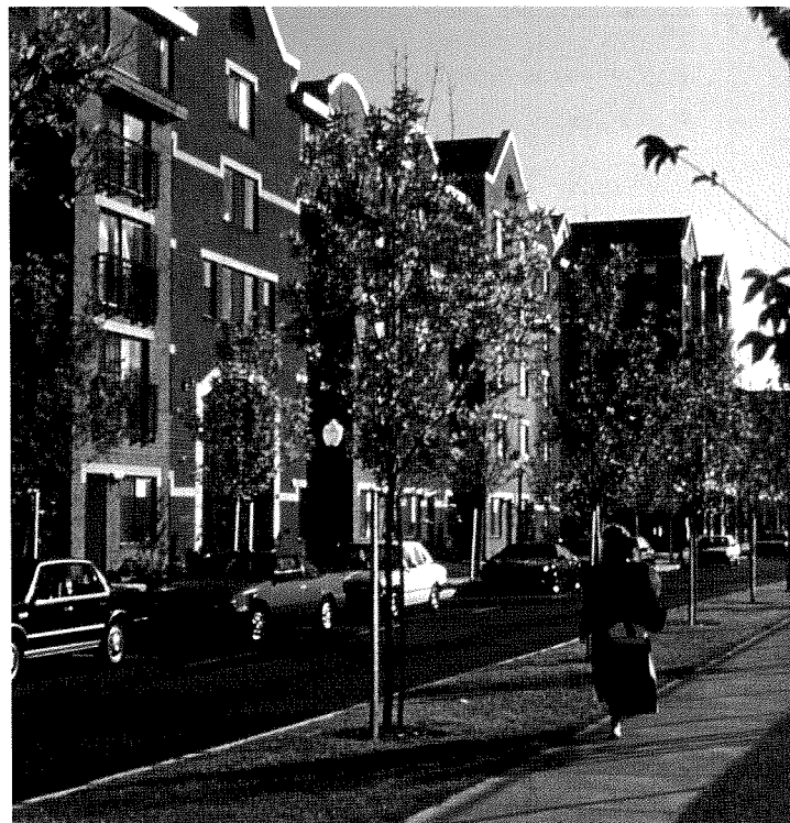
Mid-rise buildings frame Harbor Point's central mall. The first-floor units have direct private entries to the street.
