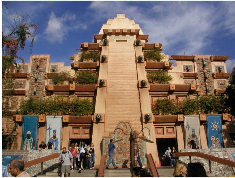
Fig. 9. Exterior of the Mexico Pavilion at EPCOT Center, Walt Disney World Florida, 2005, by Benjamin D. Esham / Wikimedia Commons, licensed under Creative Commons Attribution Share Alike CC BY 3.0 . https://en.wikipedia.org/wiki/Mexico_Pavilion_at_Epcot#/media/File:Mexico_pavilion_at_Epcot.jpg (accessed March 12, 2018).
