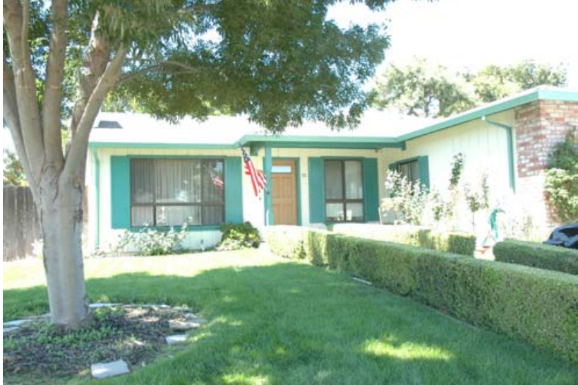
Figure 40: House 2 of the Summer 2007 test.
