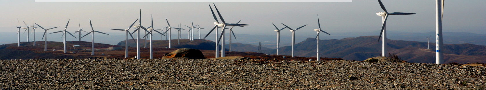
Figure 3: Mulan Wind Farm. This Mulan Wind Farm is “one of the first wind farms in China, raising the profile of renewable power and acting as a flagship for replication of the technology across the country.” It generates roughly 25 GWh of energy each year.
