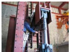
Accelerometer installed at moment-frame (UCSD)
