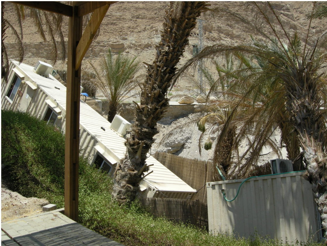
Figure 31. The destruction wrought by sinkholes at a settlement-run beach. Photo by author, 2015.
