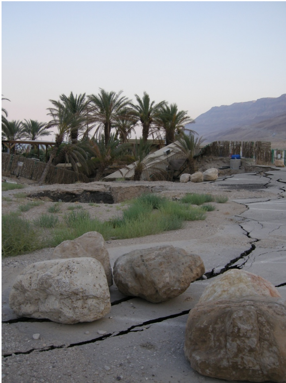
Figure 14. The destruction of the new sinkhole. Photo by author, 2015.
