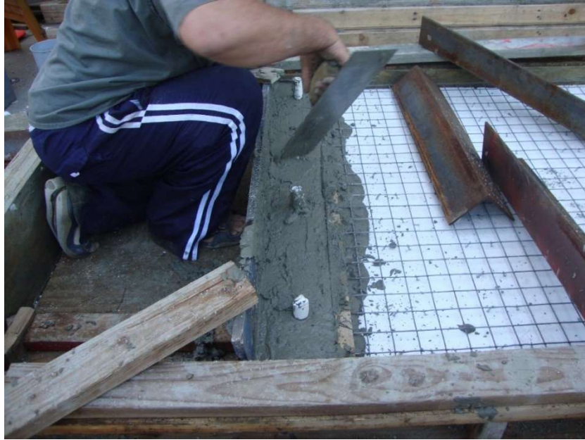
Figure (4.19): Each Side of Diagonal-CSP was filled with Mortar
