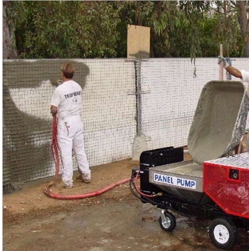
Figure (2.14): Pneumatically Application of Mortar on CSP using Hopper Spray
