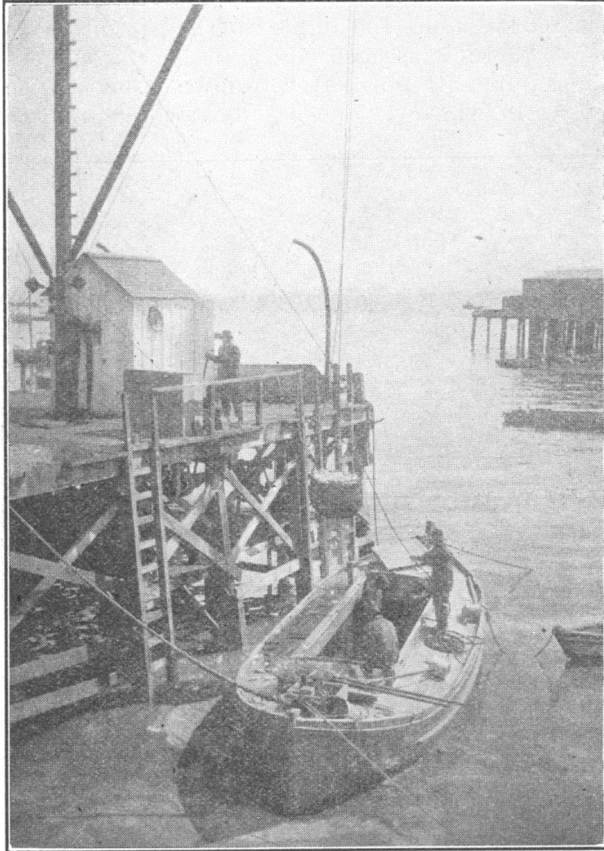
FIG. 20. Unloading sardines with "basket" hoist before the adoption of a standard metal bucket. This is not typical of Monterey in that the lighter is shown along side a wharf instead of "under the cable." Photograph by W. L. Scofield, Monterey, 1919
