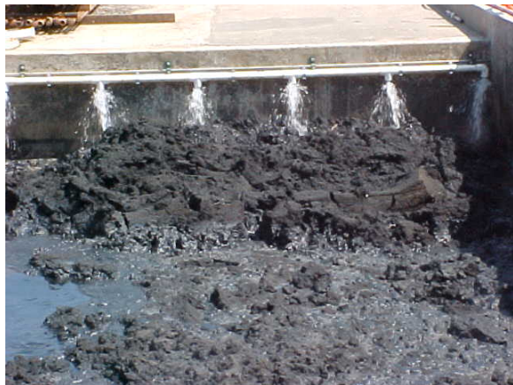
Figure 2. Biosolids in the blending pit
