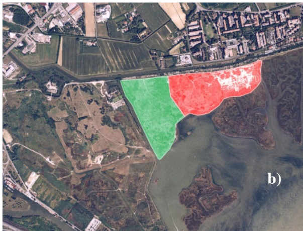
Figure 1. The Passo a Campalto dump. a) Google™ view of the Venezia Lagoon. Red box is the studied area. b) To the east are phosphogypsum (red colored), and to the west is toxic wastes (green colored).
