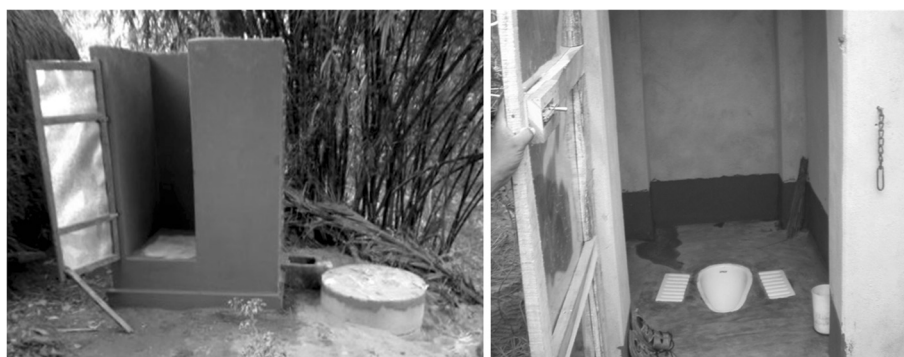
Figure 3 Photos of pour-flush latrines constructed in intervention villages (T. Clasen).
