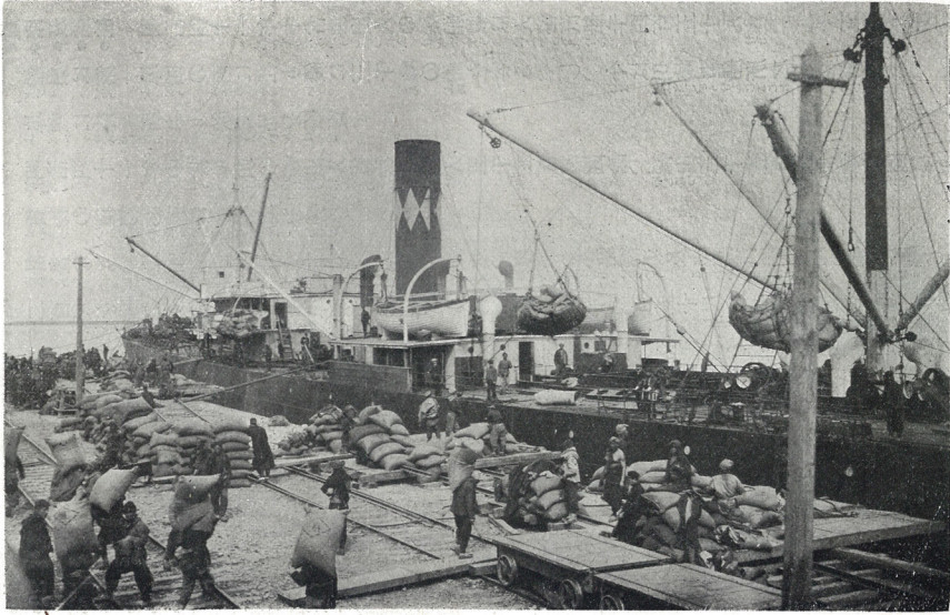
FIGURE 4. The loading of soybeans at Dairen wharf. The picture accompanied the South Manchuria Railway Company's 1909 description of Dairen wharf. It shows the three tracks of the dock railway, a ship that runs almost the length of the wharf itself, and dozens of Chinese laborers carrying and stacking hundreds of bags of soybeans. The sight to be seen was the transport of goods, not the people.
