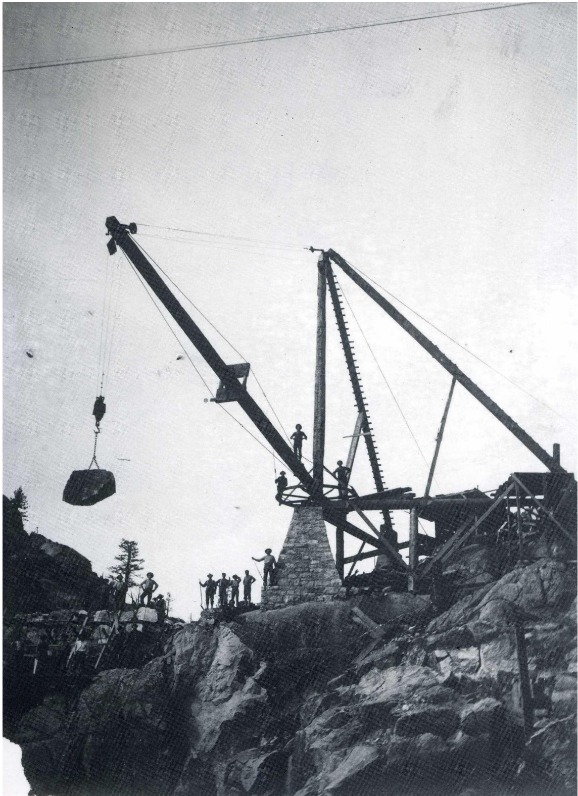
Figure 42: Construction at Relief Dam. Courtesy of Columbia Collete Library.
