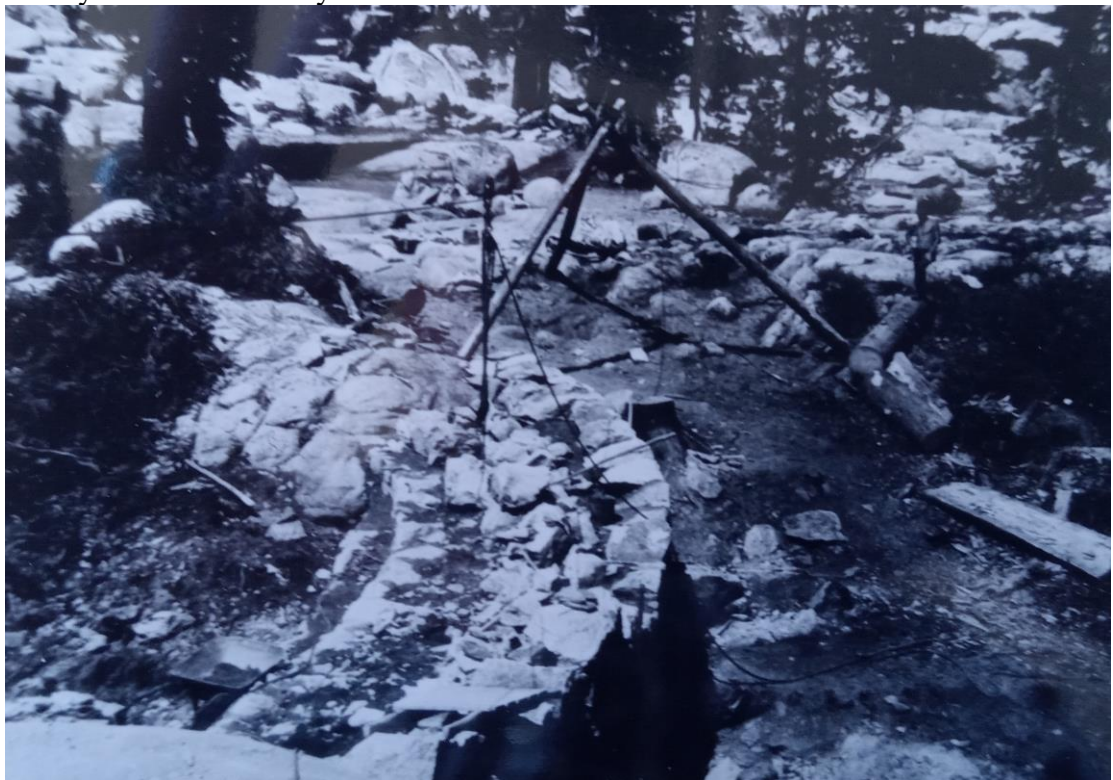
Figure 50: Civilian Conservation Corps workers constructed a check dam at Bear Lake and other similar dams, 1933. Courtesy of USDA Forest Service, Stanislaus National Forest.
