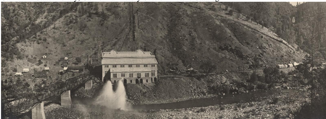
Figure 35: Stanislaus Powerhouse, ca. 1908. Courtesy of California State Library, California History Section Picture Catalog.
