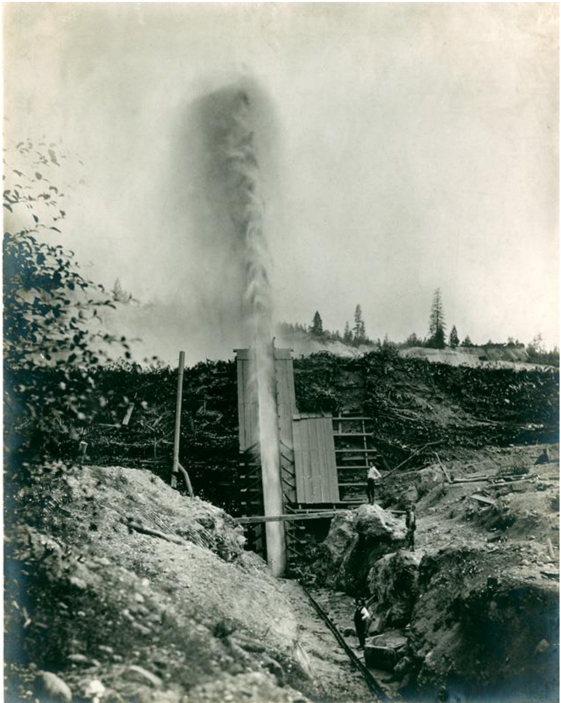
Figure 18: Hydraulic workings of the San Domingo mine, ca. 1908. Courtesy of California State Library, California History Section Picture Catalogue.
