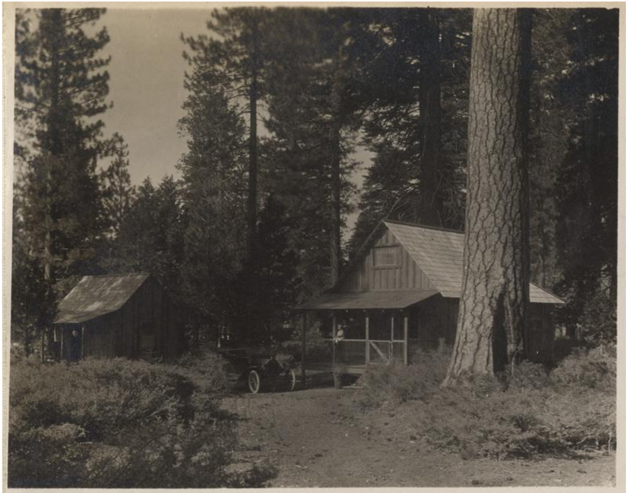
Figure 34: Camp house on Stanislaus River power system, ca. 1912-1916. Courtesy of California State Library, California History Section Picture Catalog.
