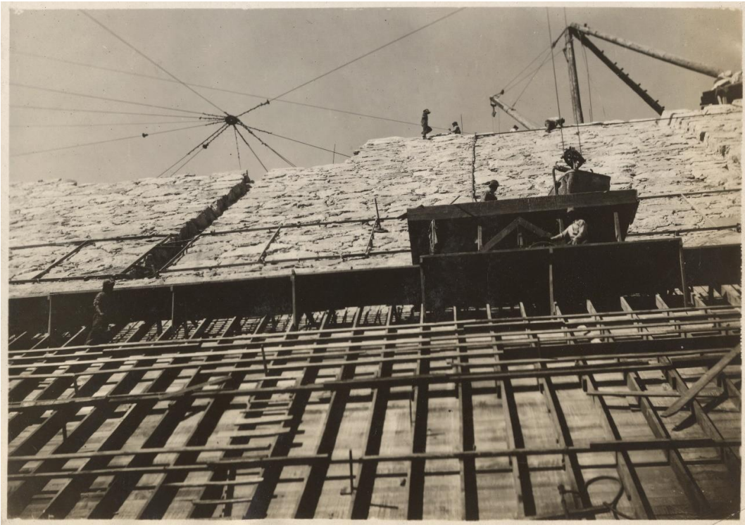
Figure 43: Construction at Strawberry Dam, 1915. Courtesy of California State Library
