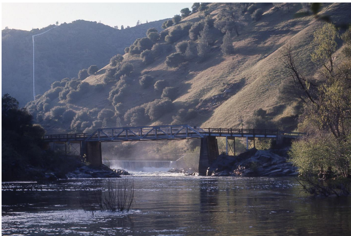
Figure 89: A crib dam and water pipe behind the put-in at Camp Nine remained in the 1970s as part of the Stanislaus power system, though major structures like the old powerhouse were gone, 1971. Larry Orman, courtesy of Stanislaus River Archive ( stanislausriver.org ).
