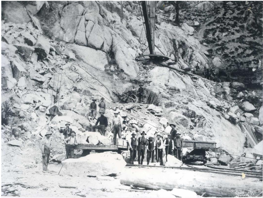
Figure 31: Workers at Relief Reservoir, ca. 1908. Courtesy of Columbia College Library.
