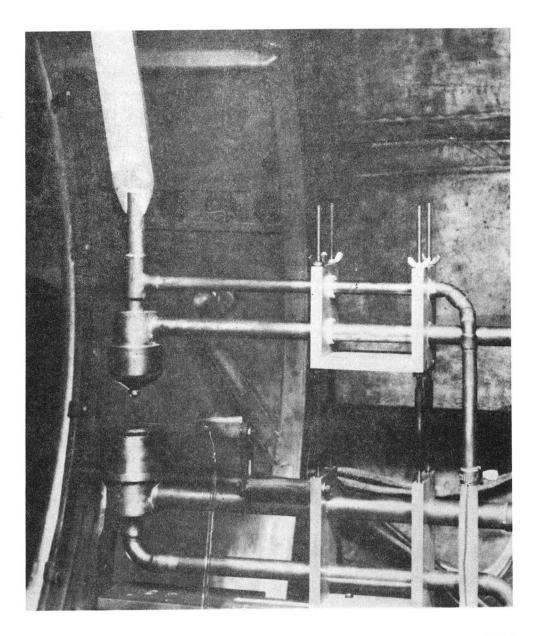
Fig. 3. Electrode configuration showing power and water leads.
