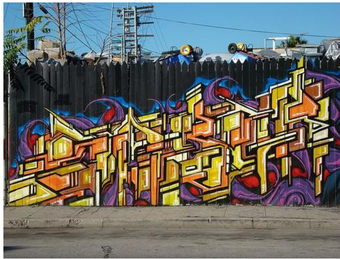
Figure 34. Wall with Graffiti . Los Angeles, California
