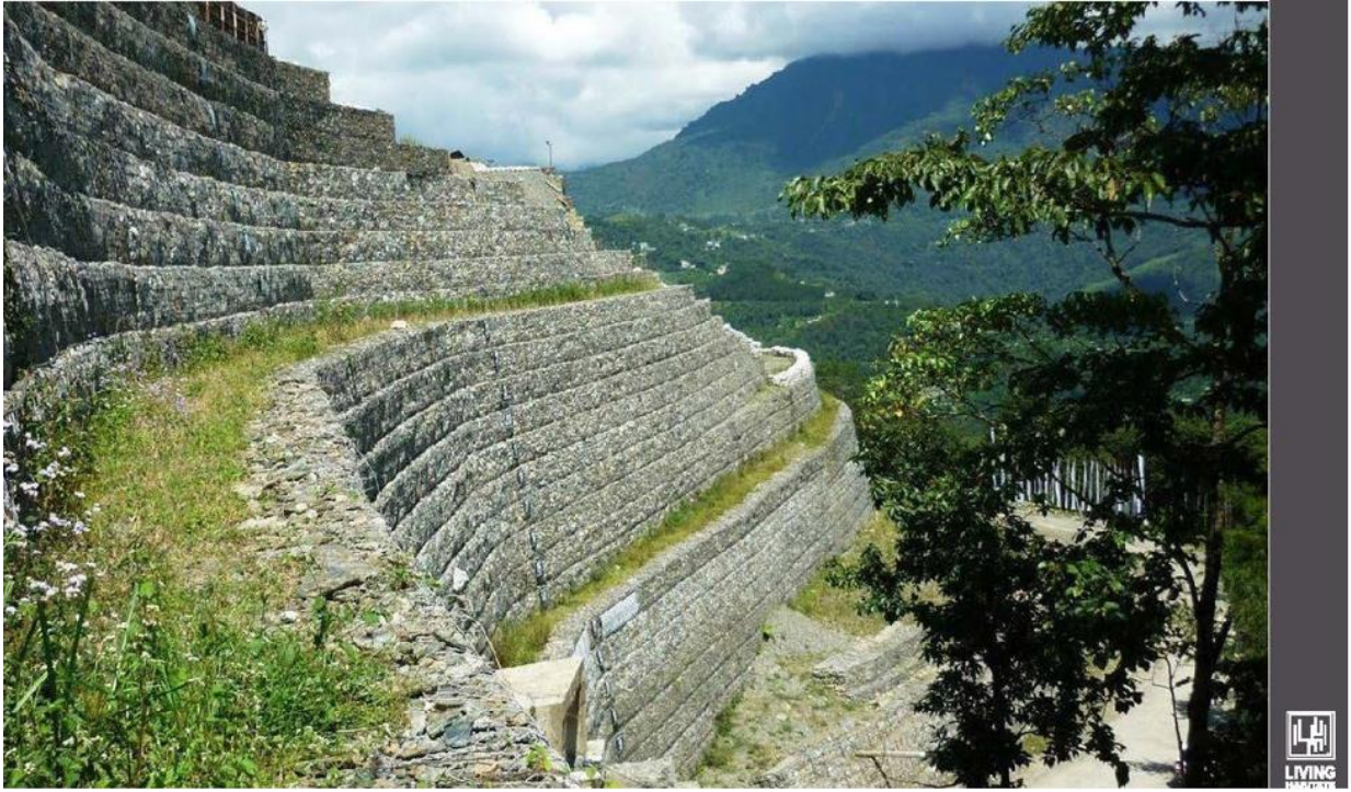
Terramesh Gabion Wall (Rock Face)
