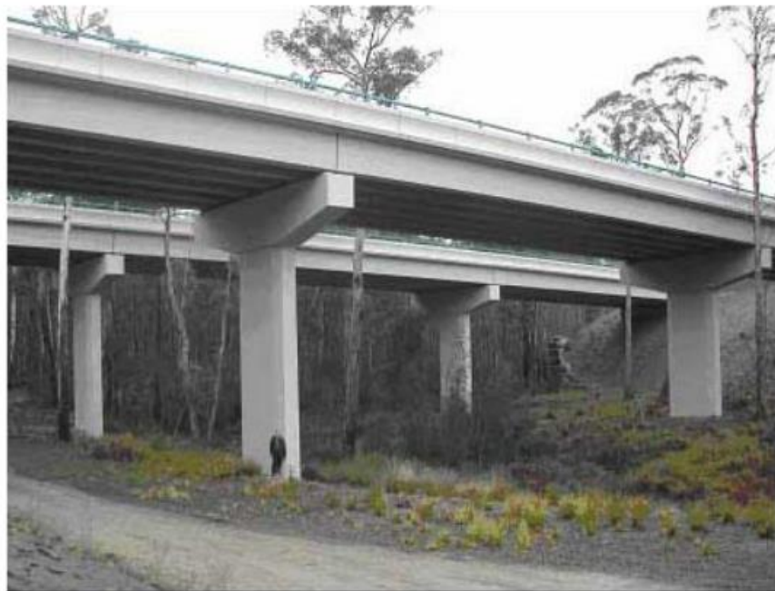
Figure 2-2: The Salty Creek Wildlife Underpass (Abson & Laurence 2003).
