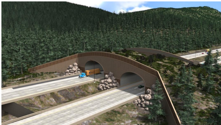
Figure 2-6: Wildlife Bridge over I-90, East of Snoqualmie Pass (Google)
