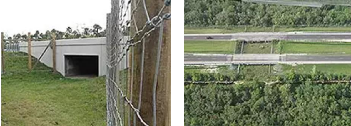
Figure 2-5: Under crossings on I-75 (Florida Fish and Wildlife Conservation Commission)
