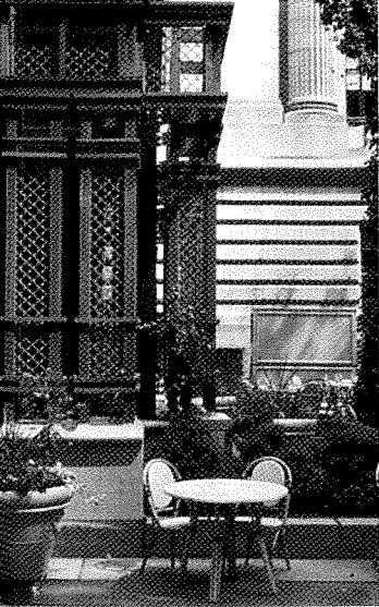
The Bryant Park Grill, a restaurant constructed along the west facade of the New York Public Library as part of the park renovation.
