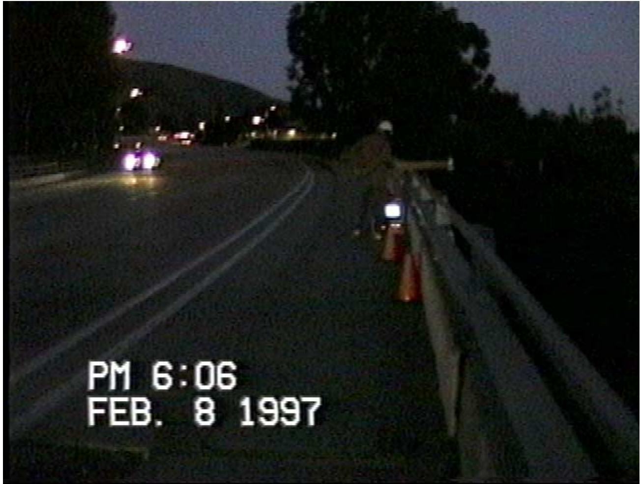
Figure 8. Typical Night Deployment of Data Acquisition System on Freeway Overcrossing.
