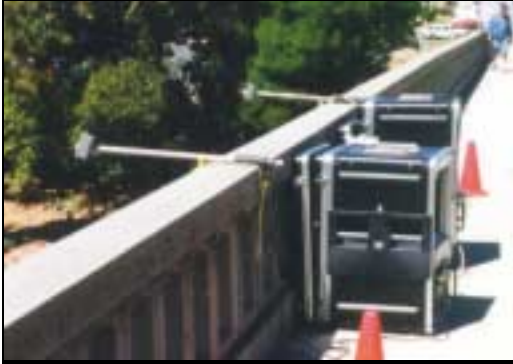
Santa Rosa St. (Hwy 1) Overcrossing
