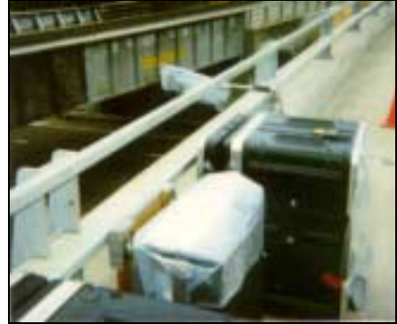
California St. (Cal Poly) Overcrossing
