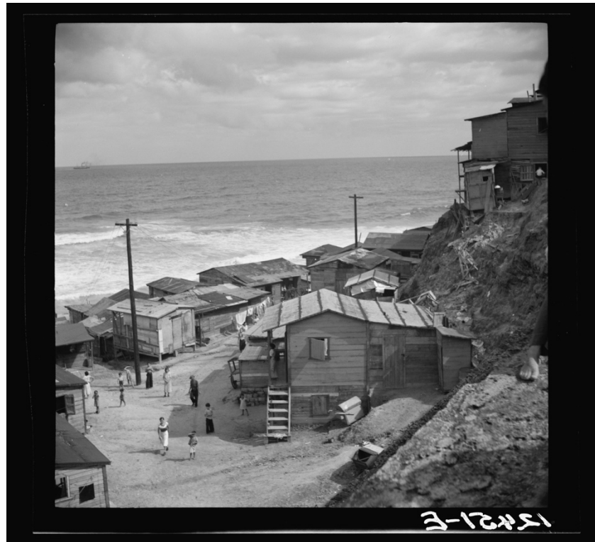
Figure 5: View of a portion of the workers' quarter of La Perla from the old Spanish ramparts, 1938, San Juan, Puerto Rico. Photo by Edwin Rosskam. Courtesy of Library of Congress, Prints & Photographs Division, Farm Security Administration/Office of War Information Black-and-White Negatives.
