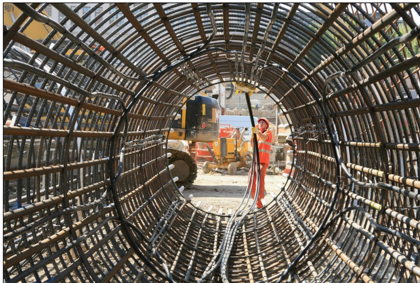
Figure 5: Full-length welded cage at One New Change London
