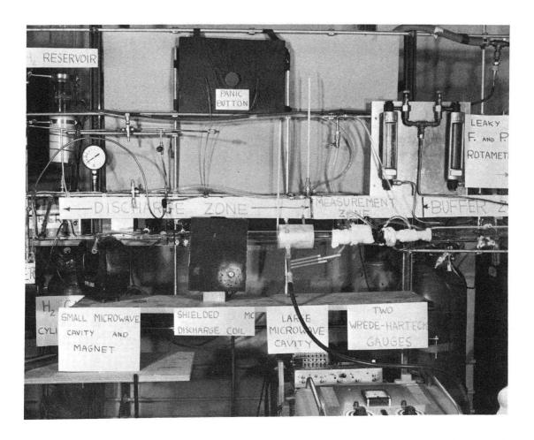
Fig. 27. Photograph of the central part of the flow-tube apparatus.
