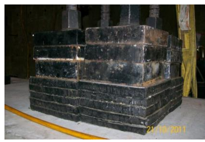
Figure 3.9 – Rubber bearing of Unit 1A: (a) components; (b) single pad; (c) assembled bearings.
