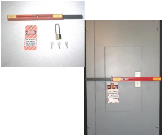
Parts for Lockout (left) and Installed Panel Lockout (right) (Electrical Panel Lockout (2017) OSHA Compliant Lockout Tagout Devices. http://www.panellockout.com/ visited by Bardaweel on 1 NOV 2017)
