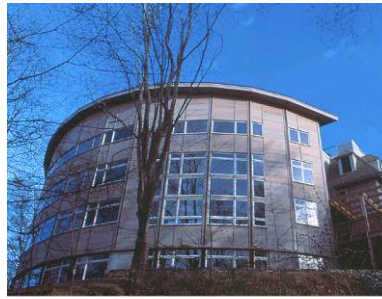
North Perspective of Office/Lab Addition Woods Hole Research Center Gilman Ordway Building
