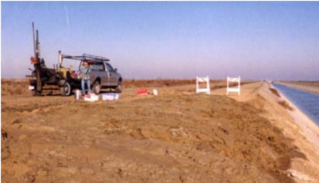
Figure C.1. Dredged SLD sediment (EP-1) drying on berm. Soil core sampling and instrument installation in progress (December 1998). View to the north.
