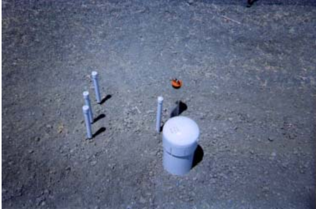
Figure C.3. Instrument cluster 7 in EP-2. From left to right: tensiometers (covered with PVC pipe), neutron probe access pipe (clear acrylic), and soil water suction lysimeters (under large PVC cap).
