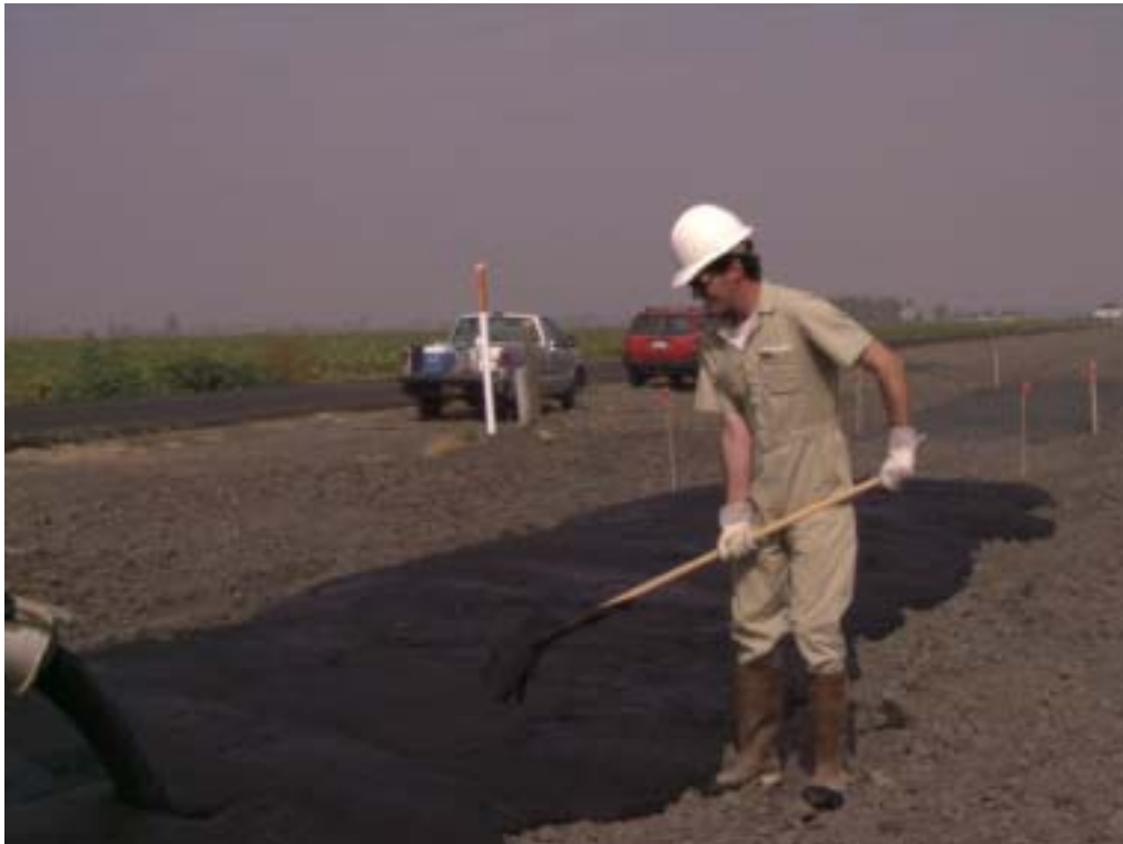
Figure C.9. Spreading of SLD sediments in FP-1 using cement rake (10/21/99)
