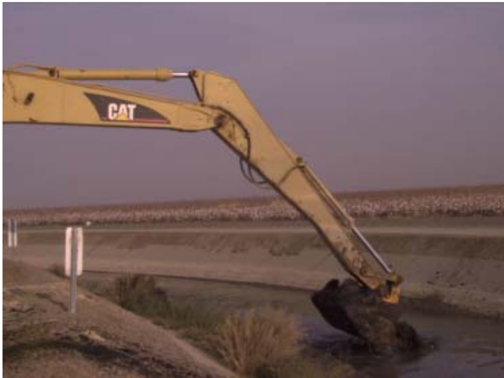
Figure C.4. Dredging of SLD sediment.
