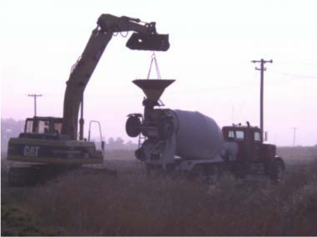
Figure C.5. SLD sediment being placed in cement truck via hopper.
