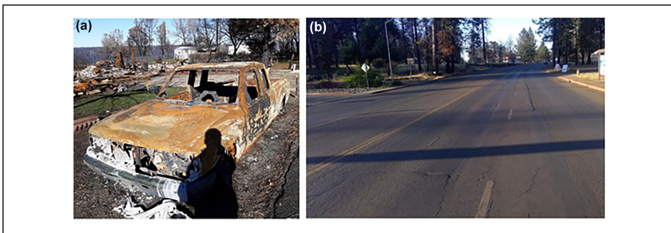
Figure 2. Town of Paradise: (a) local scarring damage from burning cars and (b) fatigue and rutting of Skyway in Paradise City.
