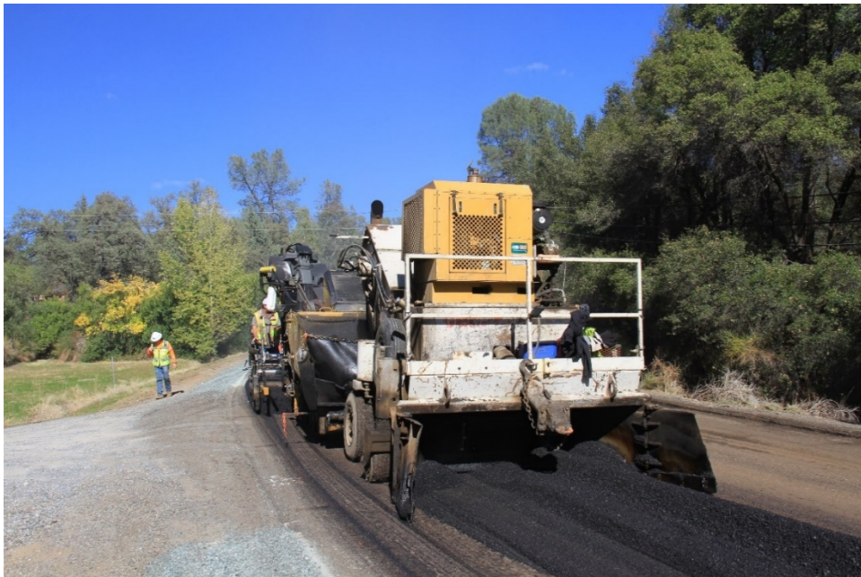
Figure 5.5: Windrow pick up of a mix containing RAS.
