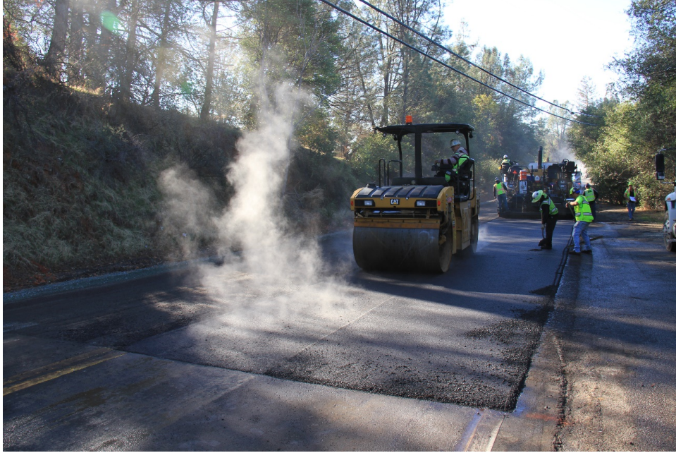
Figure 5.8: Breakdown rolling.
