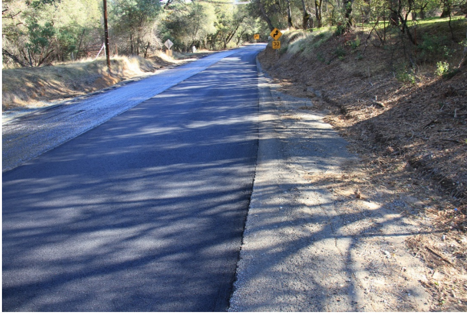
Figure 5.6: One lane paved with a mix containing RAS (Mix C) and other lane with tack coat before overlay.
