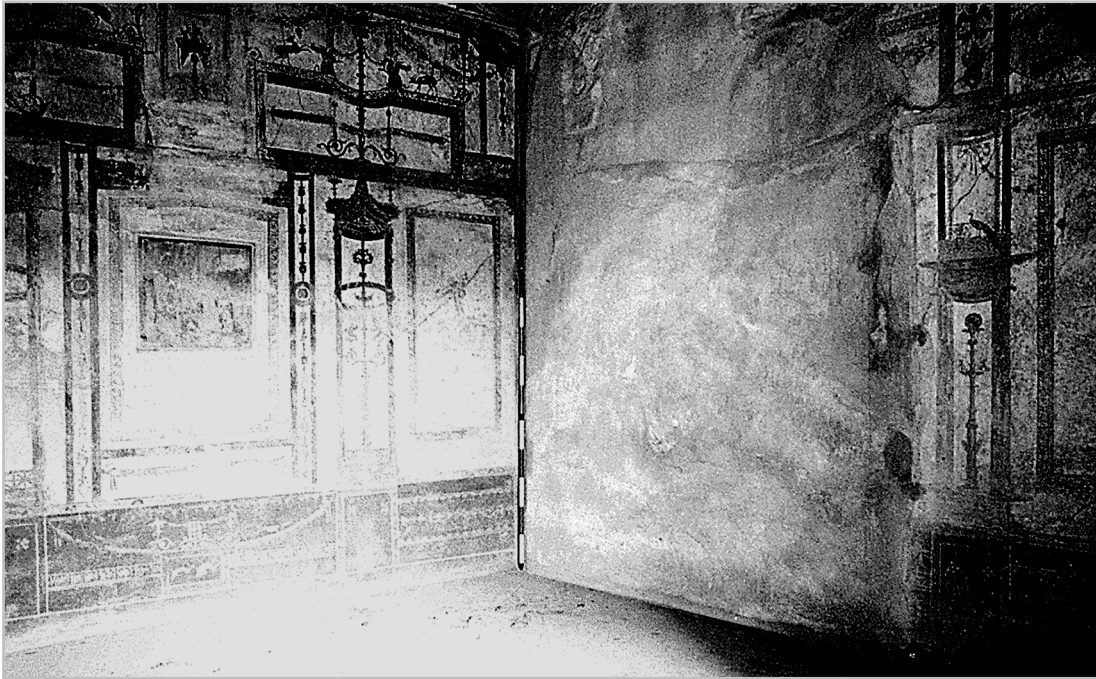
Figure 2.6 Coarsely plastered area of south wall, room k, Casa del Principe di Napoli
