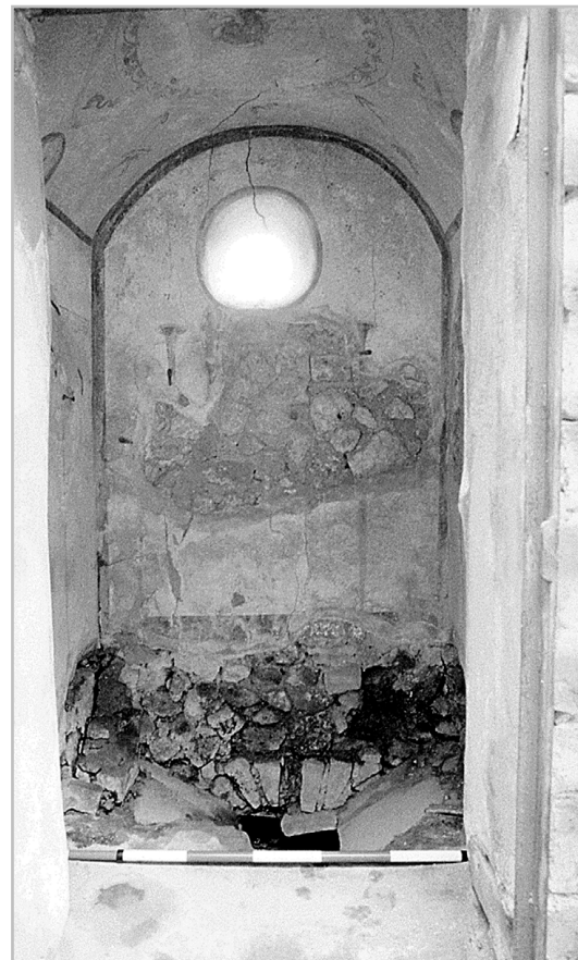
Figure 5.13 Painted walls and ceiling, latrine s1, Casa delle Nozze d'Argento
