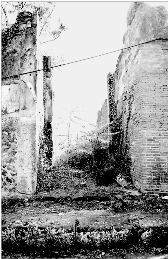
Figure 3.3 House VIII 2,34 overgrown with vegetation
