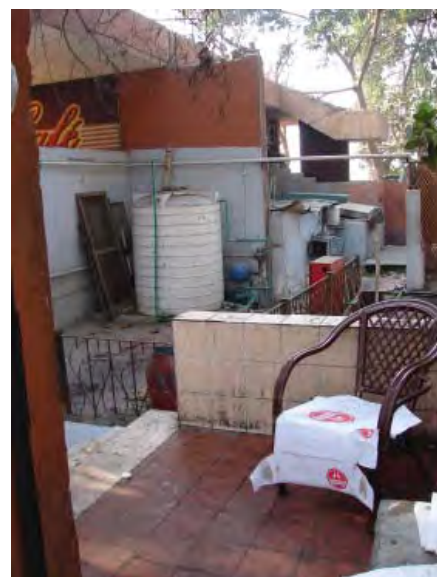
FIGURE 10. Blocked access Ventilation units and storage facilities for private clubs prevent pedestrian access to the Nile waterfront from the sidewalk.
