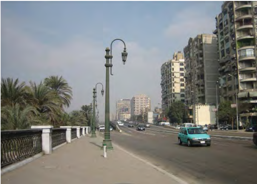
FIGURE 70. Vehicular overpass on the Corniche
