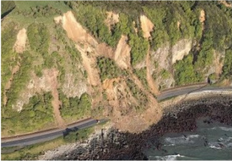
Figure 2: Landslide blocking the railway line and State Highway 1 north of Kaikōura. The landslide has broken the railway line and dragged the tracks across the road on the right hand side of the photo. The coastal uplift at this site is also visible in the exposed shoreline covered with sub-tidal seaweed. (Photo: S. Dellow 14/11/2016).
