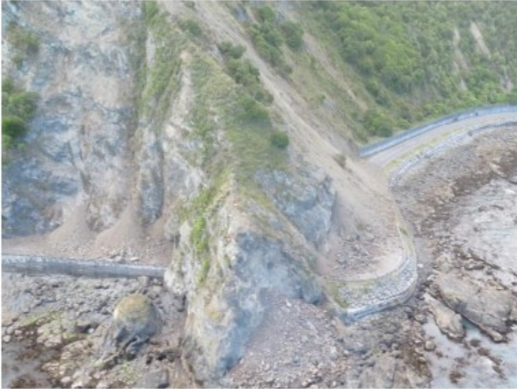
Figure 3: Landslides on either side of the Paratatahi Tunnels, State Highway 1, south of Kaikōura. The railway line at this location is enclosed in a rock shelter, and so was not directly affected. (Photo: S. Cox, 20/11/2016).
