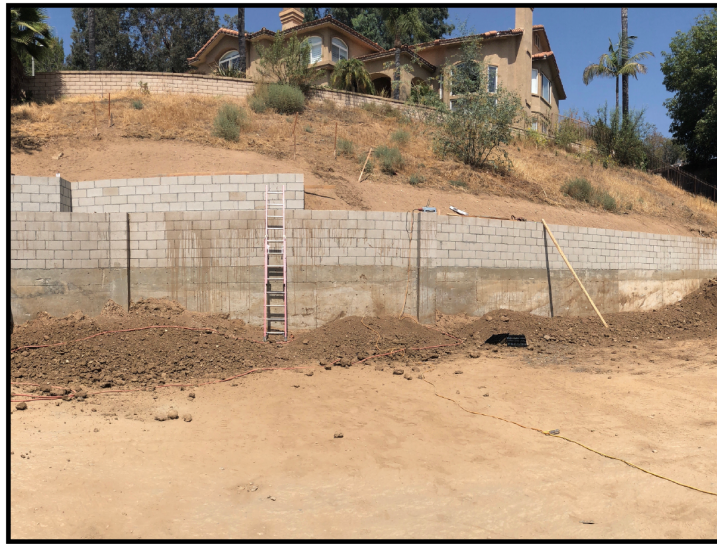
Figure 2.1: A cantilever retaining wall constructed of concrete masonry units (CMU) and Portland Cement Concrete (PCC)
